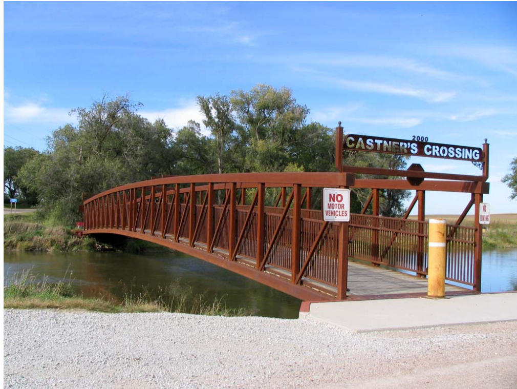
Photo E-40. Castner’s Crossing footbridge, which crosses the Loup Power Canal and connects the Two Lakes Trail and the Bob Lake Trail.
