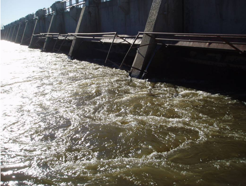
Photo E-4. Downstream face of the Intake Gate Structure.
