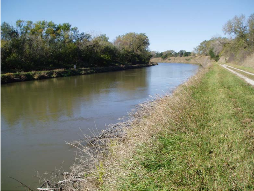
Photo E-43. View of the Upper Power Canal.
