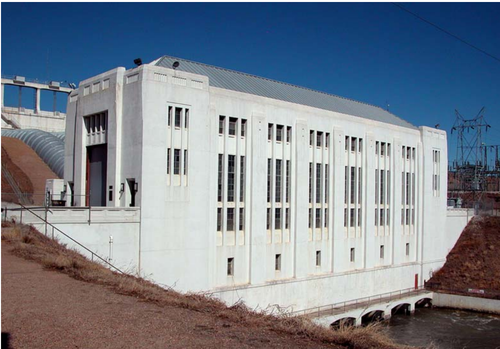
Photo E-55. The art deco style of the Columbus Powerhouse.
