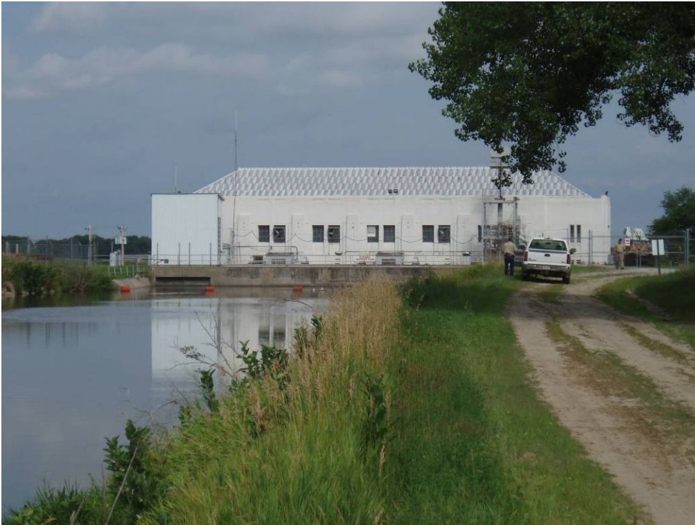
Photo E-12. View of the upstream face of the Monroe Powerhouse; the flow bypass gate is located inside the enclosure at left.
