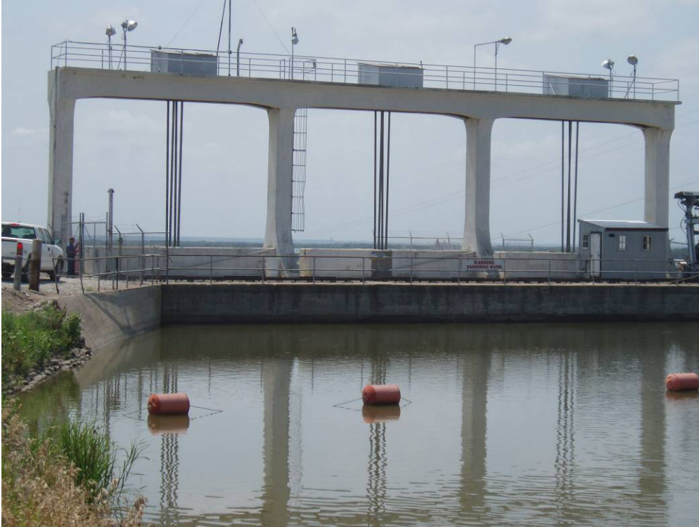
Photo E-18. Upstream face of the Powerhouse Inlet Structure.
