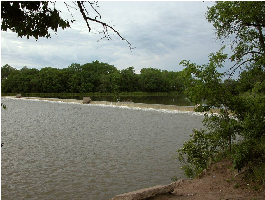
Photo E-49. View of the Outlet Weir from the east bank.
