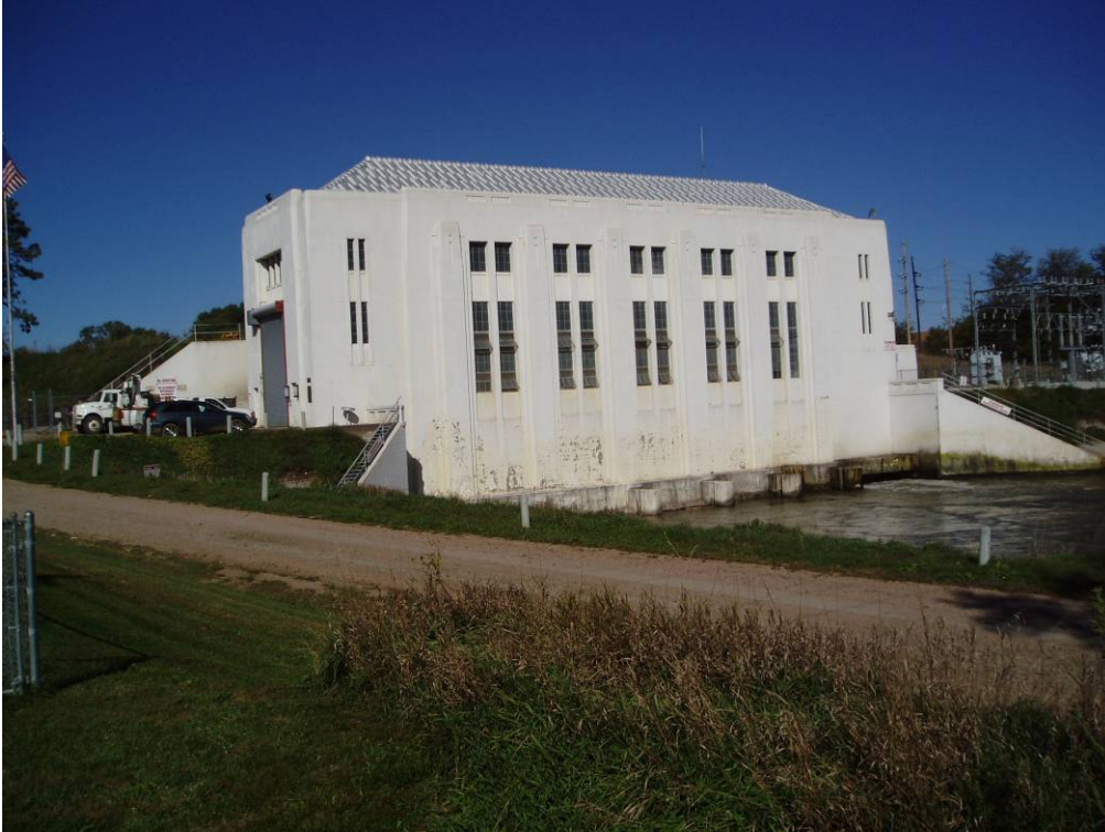
Photo E-13. View of the downstream face of the Monroe Powerhouse.
