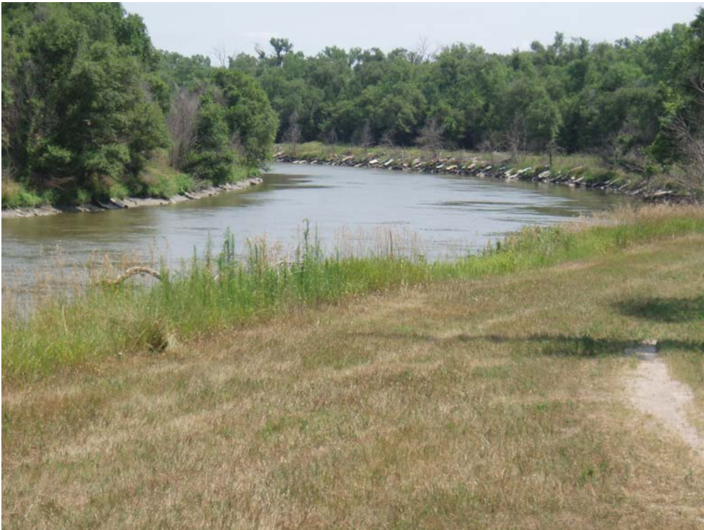
Photo E-47. View of the Tailrace Canal.
