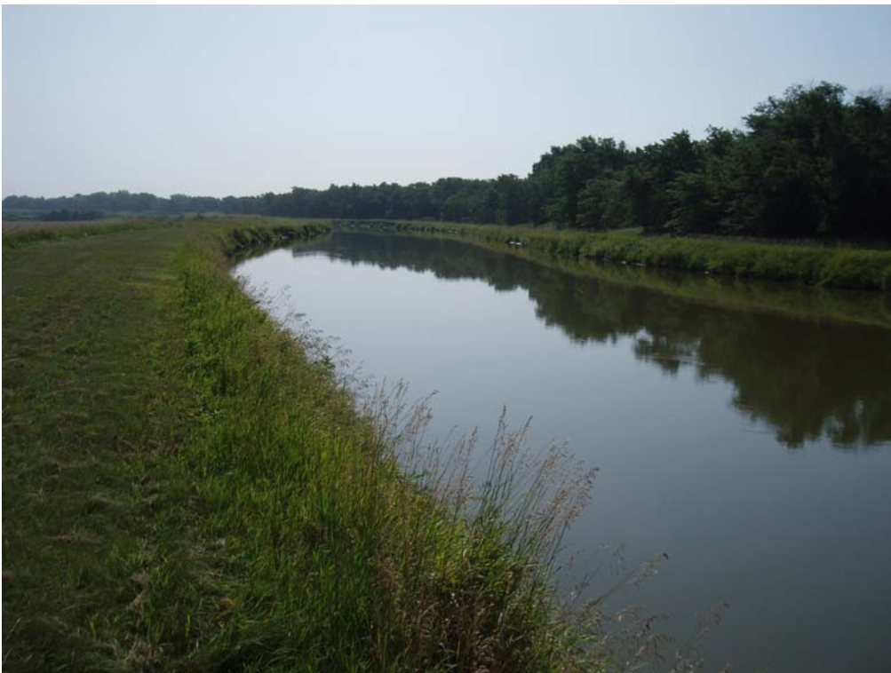
Photo E-45. View of the Lower Power Canal.
