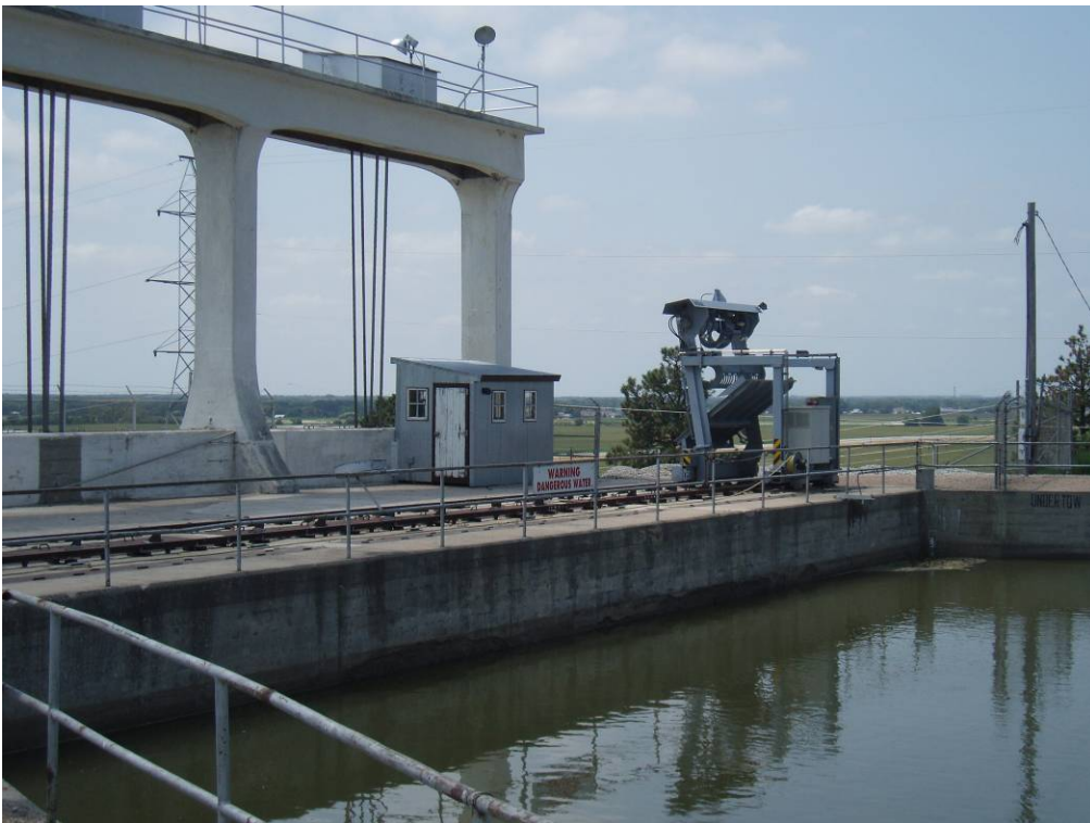
Photo E-19. Operating deck of the Powerhouse Inlet Structure.
