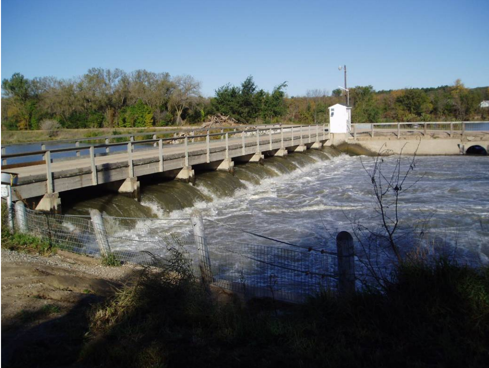
Photo E-9. View of flow exiting the Skimming Weir.
