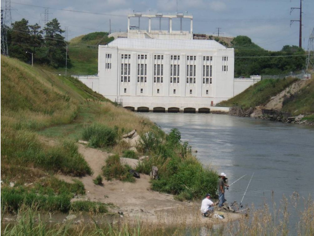
Photo E-22. View of the Columbus Powerhouse from the Tailrace Canal.
