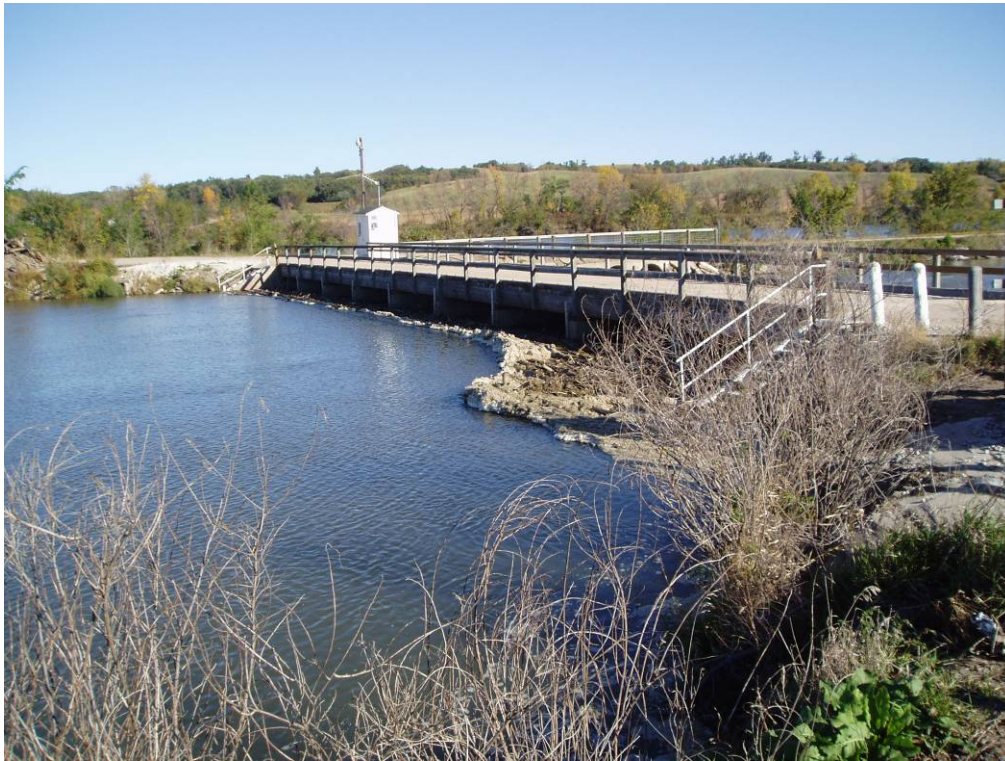
Photo E-8. View of the Skimming Weir from upstream.
