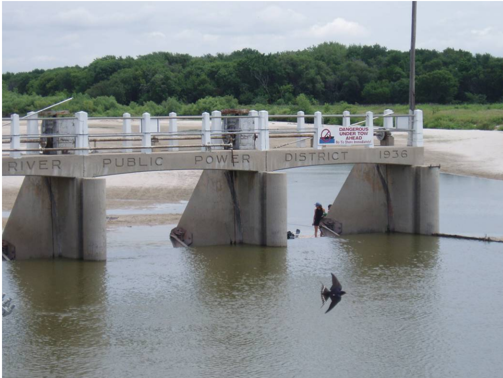
Photo E-5. Upstream face of the Sluice Gate Structure.
