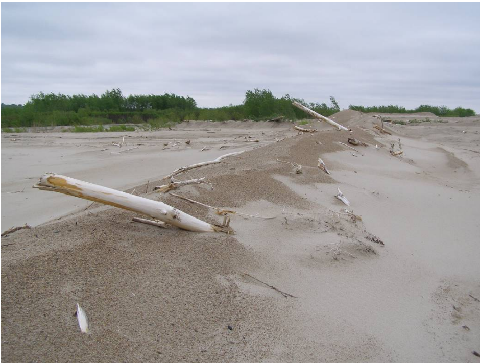
Photo E-31. Protective berm in 2008; limbs and branches stabilize sand.
