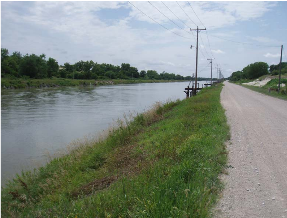
Photo E-51. View of the Settling Basin and an access road.
