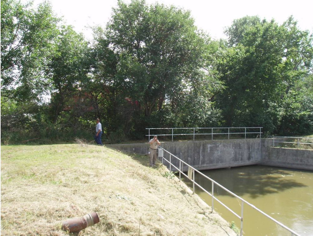
Photo E-11. View of the Railroad Siphon exit.
