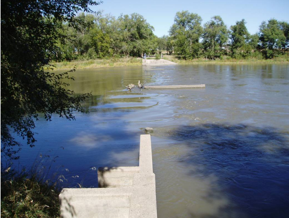
Photo E-15. Unique turbulence created by the submerged Sawtooth Weir.
