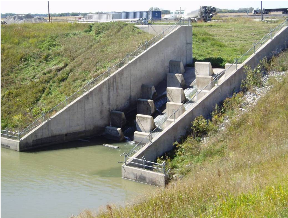
Photo E-23. View of the Lost Creek Flood Control Channel spillway.
