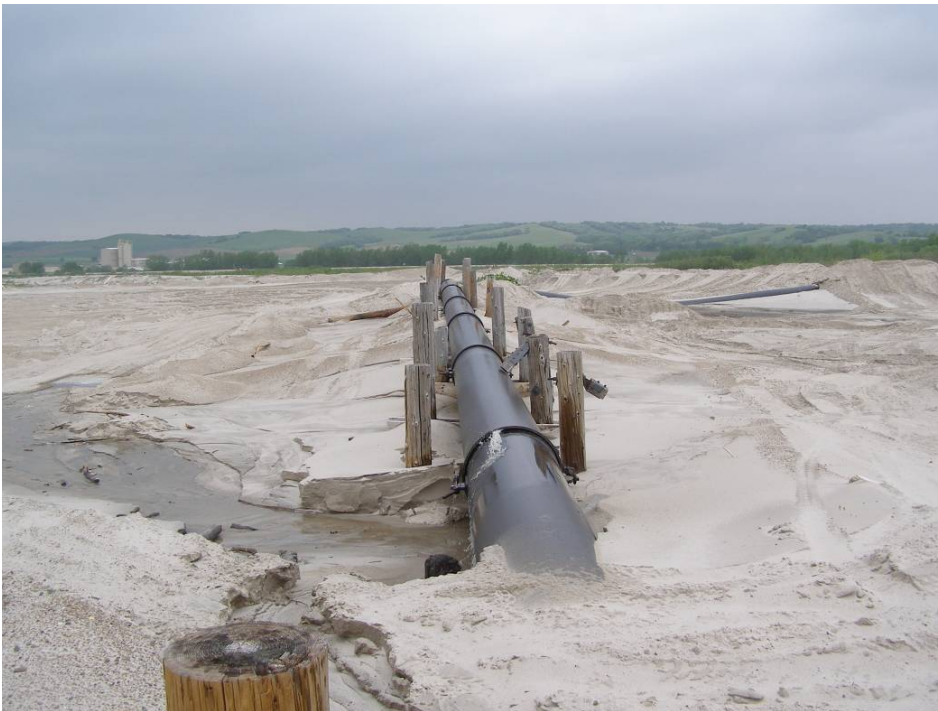
Photo E-33. Discharge pipe extension to divert water around berm in 2008.
