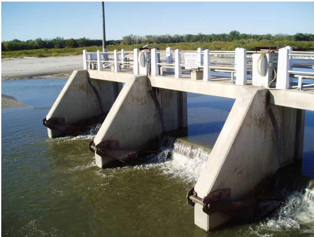
Photo E-6. Downstream face of the Sluice Gate Structure.
