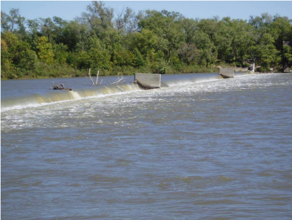
Photo E-24. View of the Outlet Weir from the west bank.
