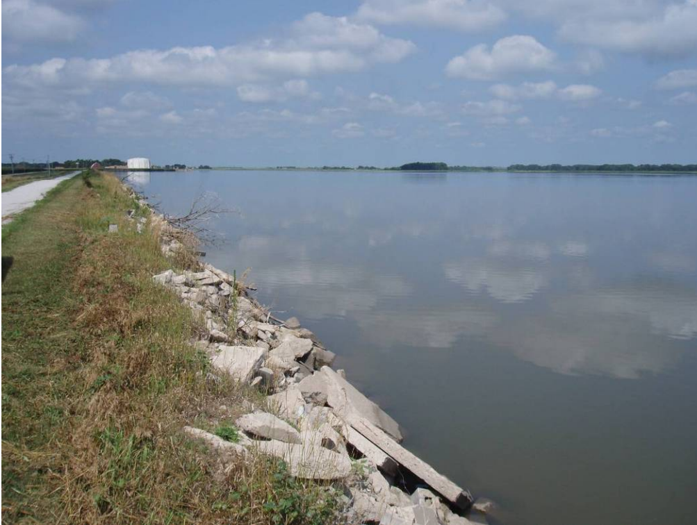
Photo E-25. Riprap shore protection on Lake Babcock.
