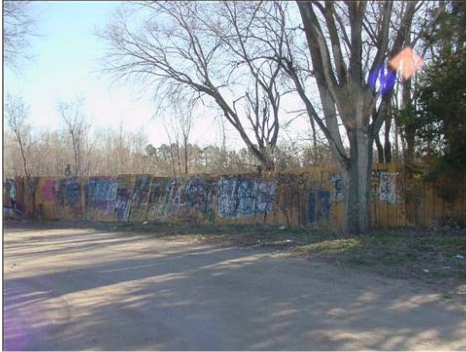
Photo 2. Vandalism at Tailrace Park: photographed April 5, 2011.
