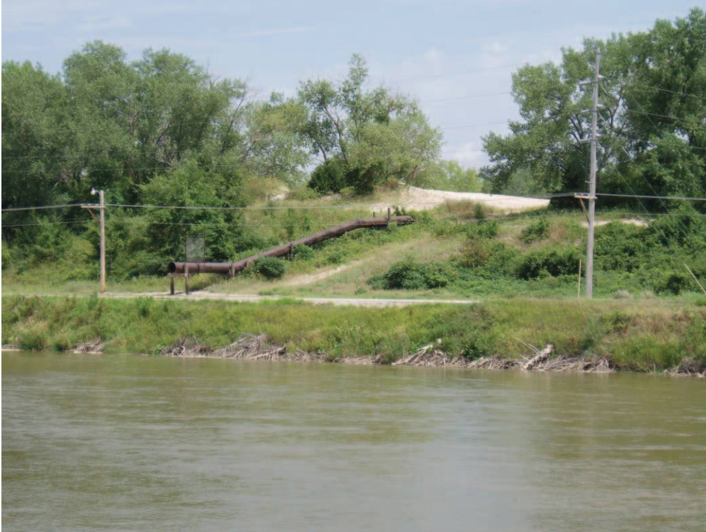
Photo 4. Typical discharge piping and shoreline stabilization at the South Sand Management Area.
