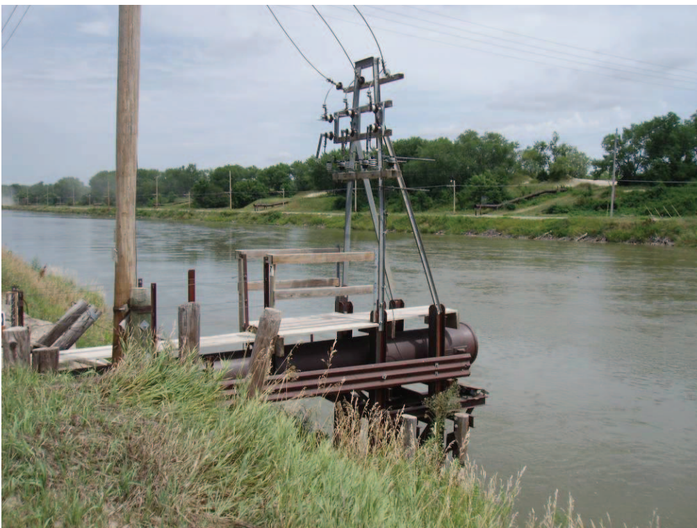
Photo 3. A typical dredge connection point along the Settling Basin.
