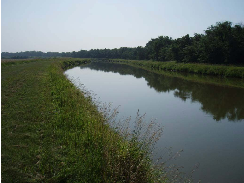
Photo 3. Typical view of the Lower Power Canal.
