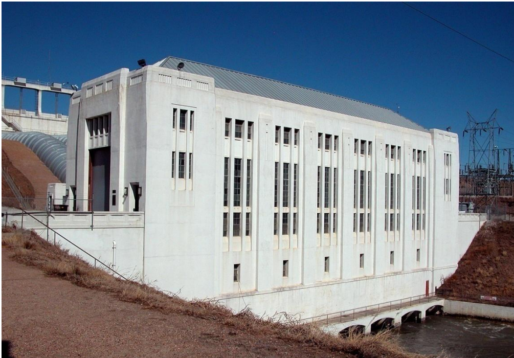
Photo 12. View of the Columbus Powerhouse from the Tailrace Canal.
