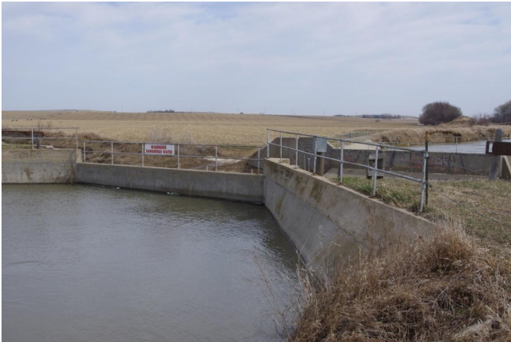
Photo 16. View of the Dry/Cherry Creek Siphon inlet.
