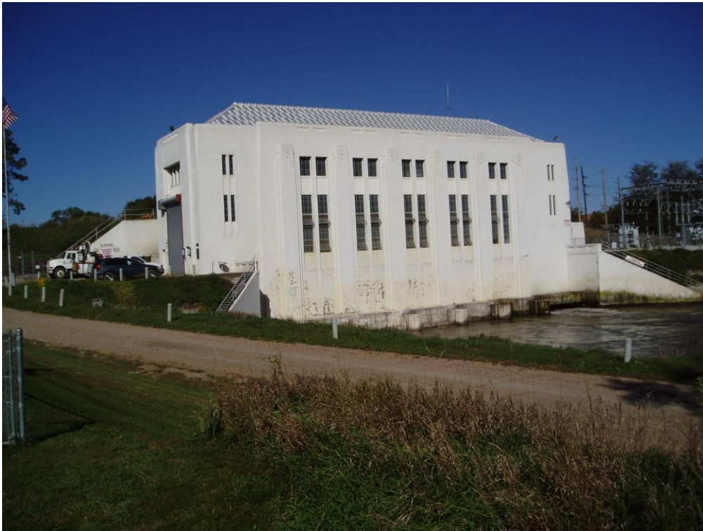
Photo 11. View of the downstream face of the Monroe Powerhouse.
