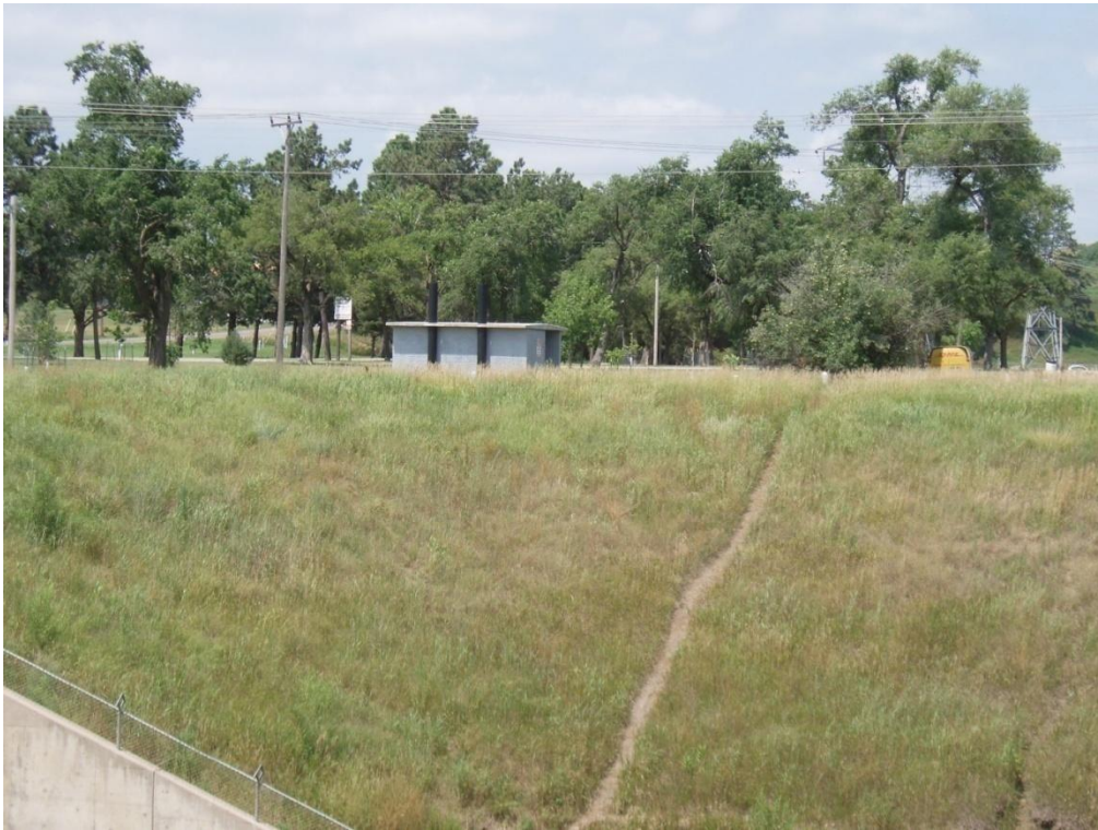
Photo 7. Columbus Powerhouse Park facilities.
