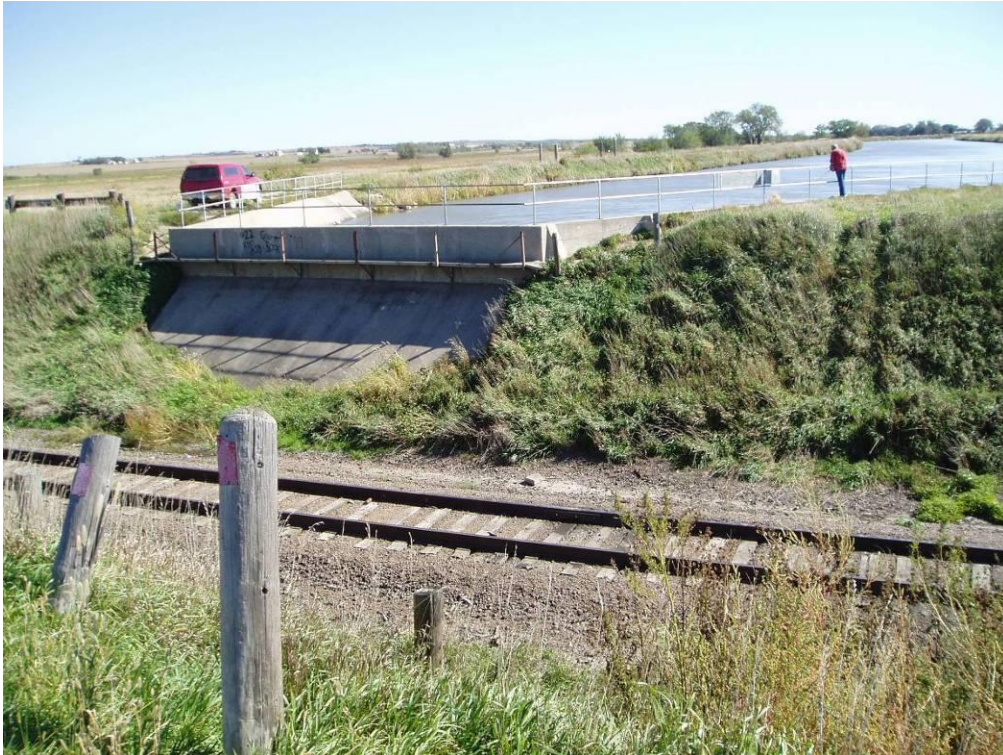
Photo 17. View of the Lower Power Canal at the Oconee Siphon.
