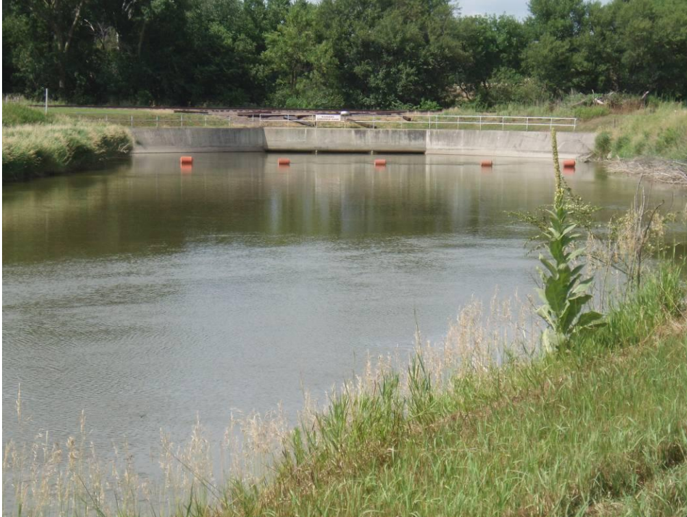
Photo 14. View of the approach to the Railroad Siphon at Genoa.
