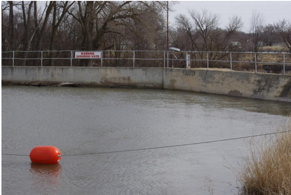
Photo 13. View of the Beaver Creek Siphon.
