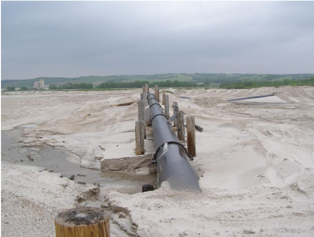
Photo 10. Typical view of the North Sand Management Area.
