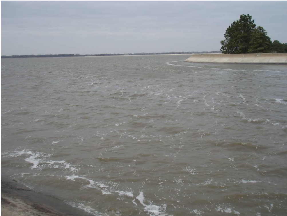
Photo 3. View of Lake Babcock from the south dike at the outlet.
