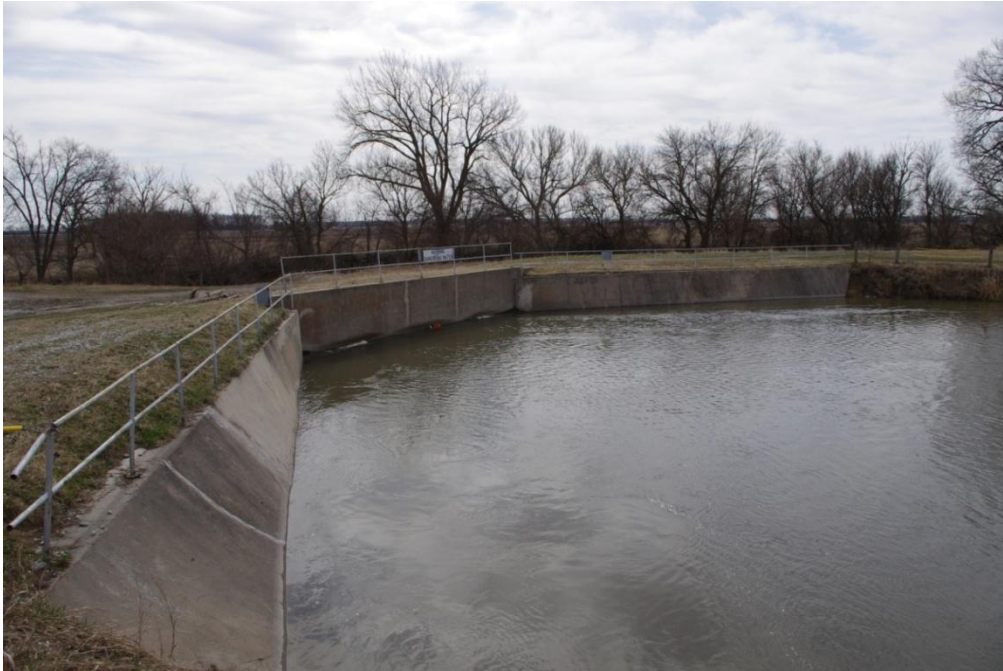
Photo 15. View of the Looking Glass Creek Siphon.
