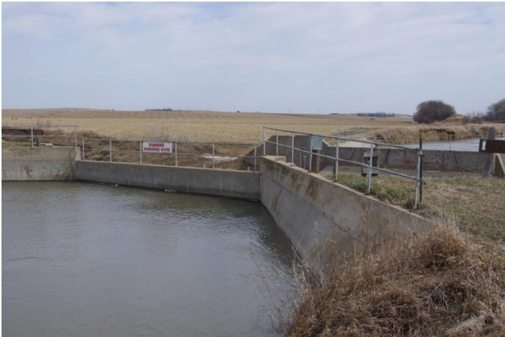
Photo 16. View of the Dry/Cherry Creek Siphon inlet.
