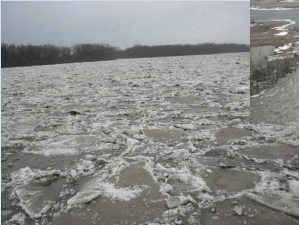
2010 Ice Jam at N-39 Bridge
