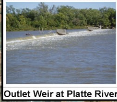
Outlet Weir at Platte River
