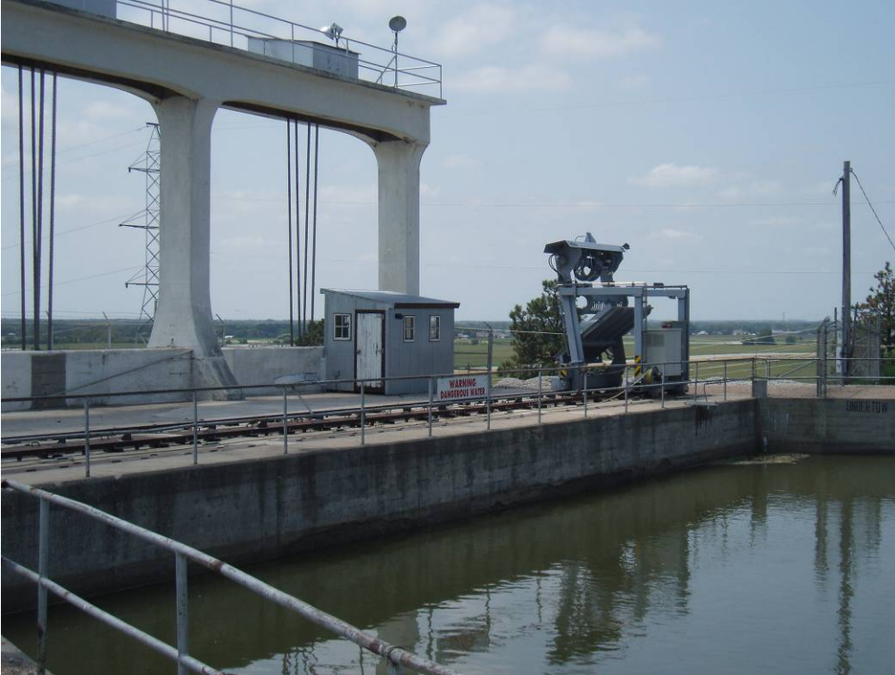
Photo 4-34. Operating deck of the Powerhouse Inlet Structure.
