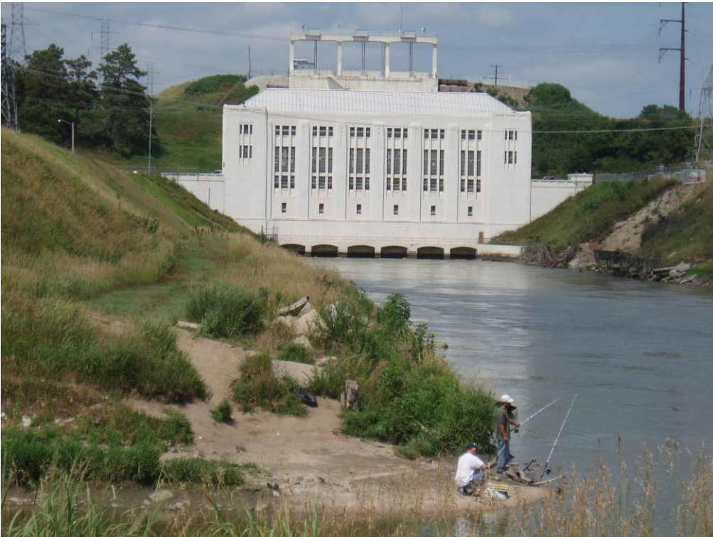
Photo 4-37. View of the Columbus Powerhouse from the Tailrace Canal.
