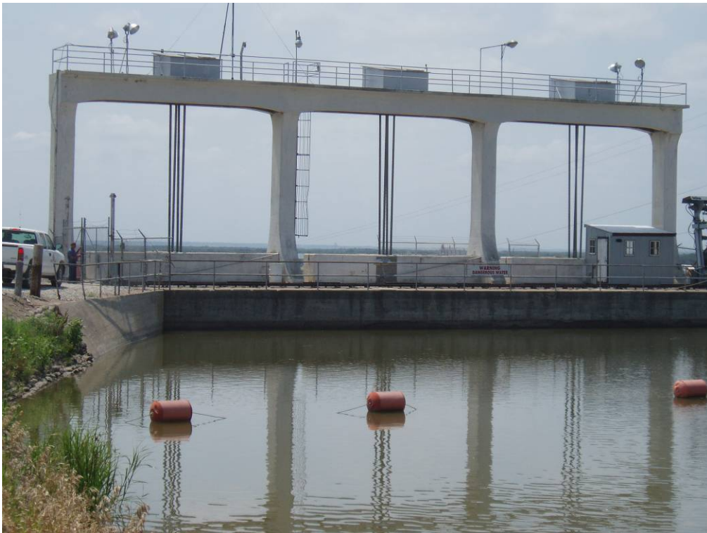
Photo 4-33. Upstream face of the Powerhouse Inlet Structure.
