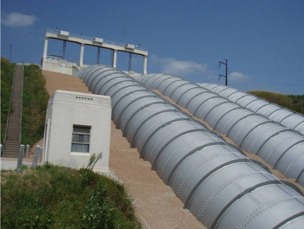
Photo 4-35. View of the Penstocks from the Columbus Powerhouse.
