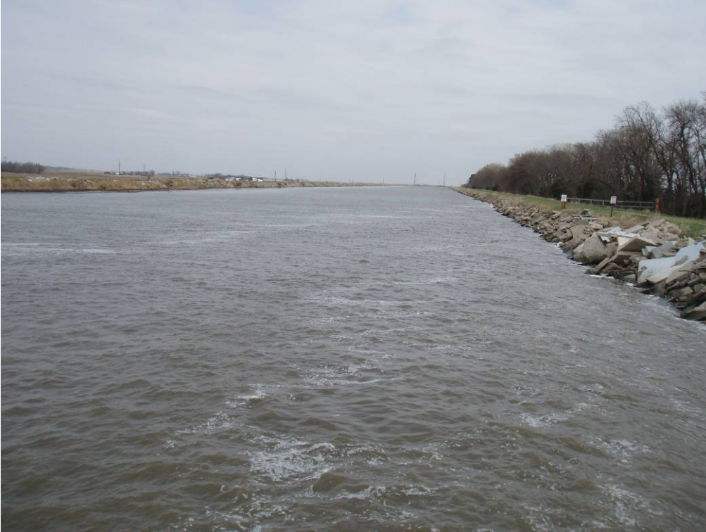
Photo 4-31. View of the Intake Canal as it exits Lake Babcock.
