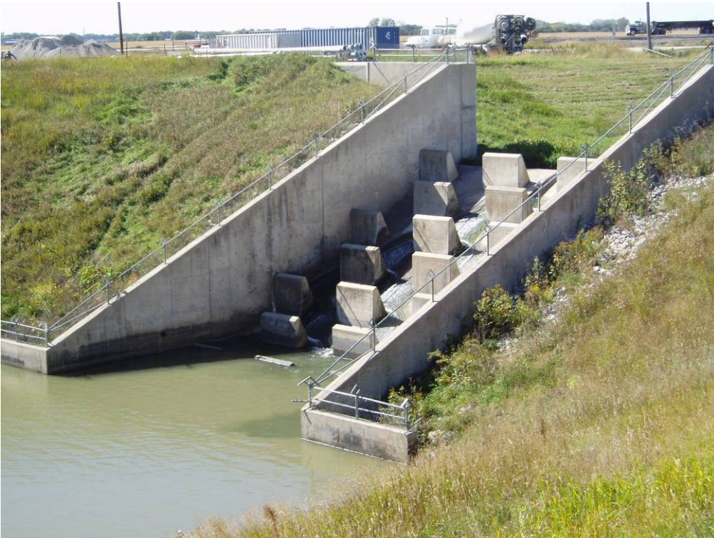
Photo 4-39. View of the Lost Creek Flood Control Channel spillway.
