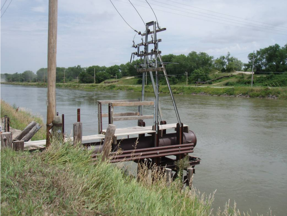
Photo 4-11. A typical dredge connection point along the Settling Basin.
