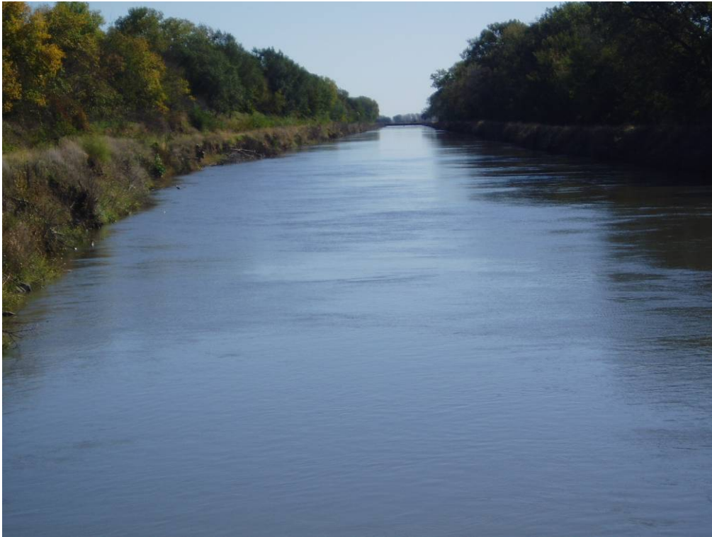
Photo 4-17. Typical view of the Upper Power Canal.
