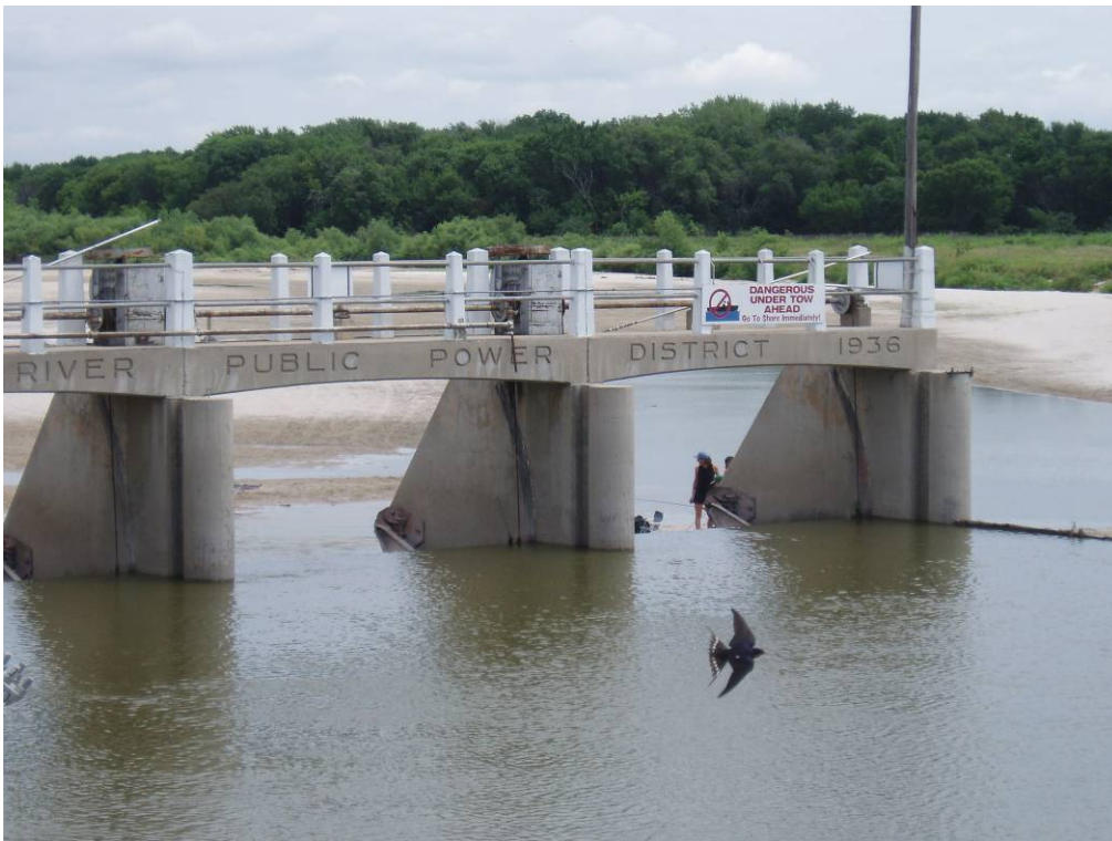
Photo 4-5. Upstream face of the Sluice Gate Structure.
