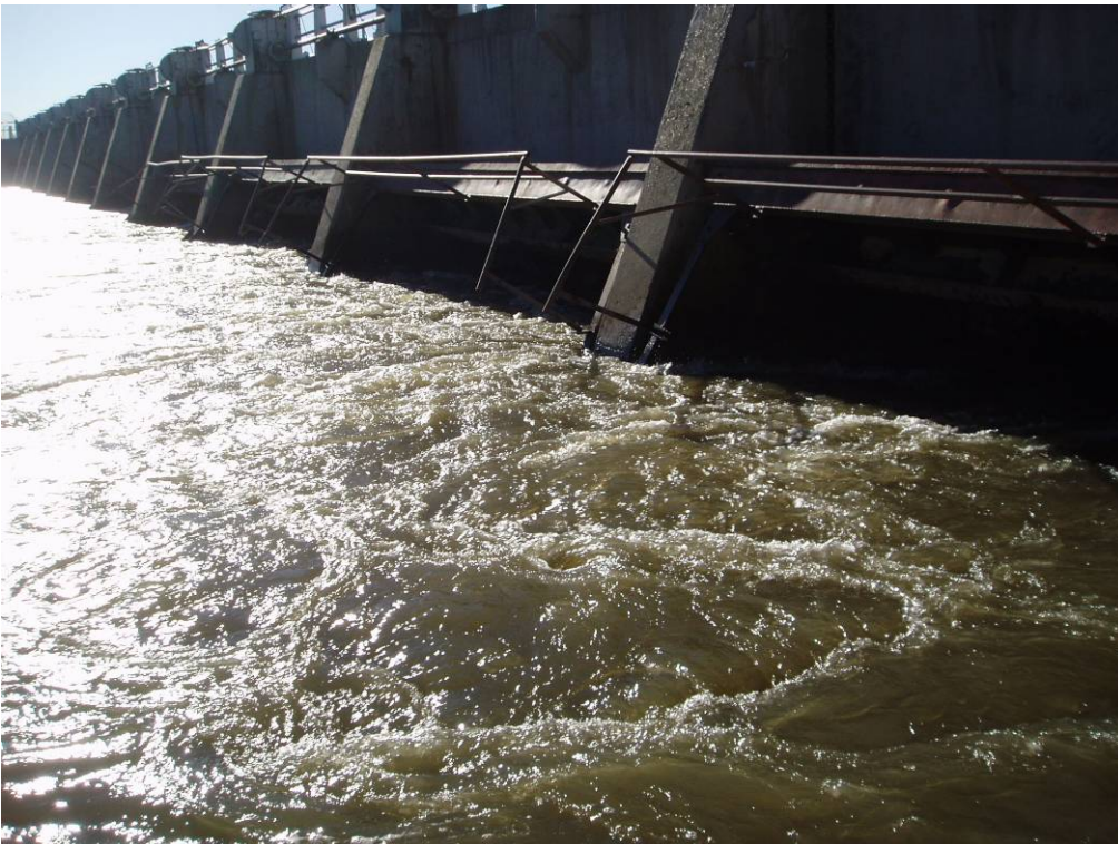
Photo 4-4. Downstream face of the Intake Gate Structure.
