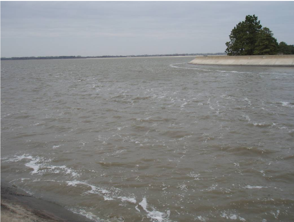
Photo 4-28. View of Lake Babcock from the south dike at the outlet.
