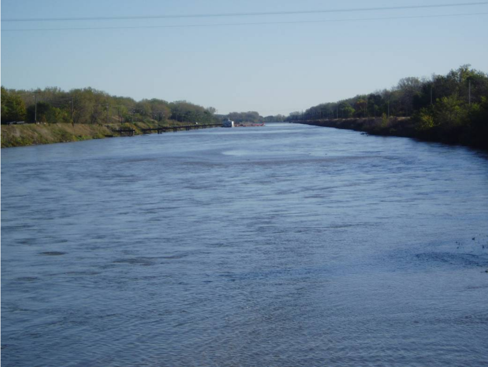
Photo 4-7. View of the Settling Basin from the Intake Gate Structure.
