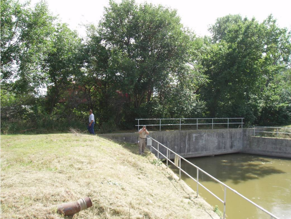
Photo 4-20. View of the Railroad Siphon exit.
