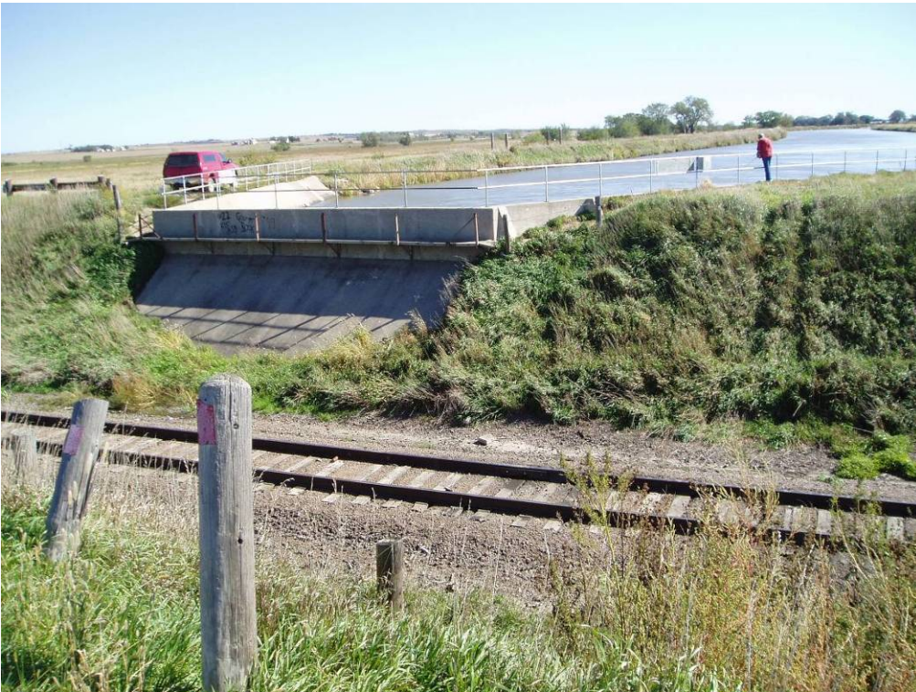
Photo 4-24. View of the Lower Power Canal at the Ocone Siphon.
