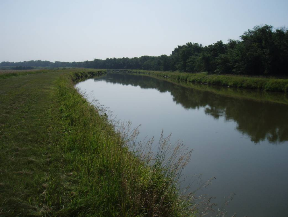
Photo 4-23. Typical view of the Lower Power Canal.
