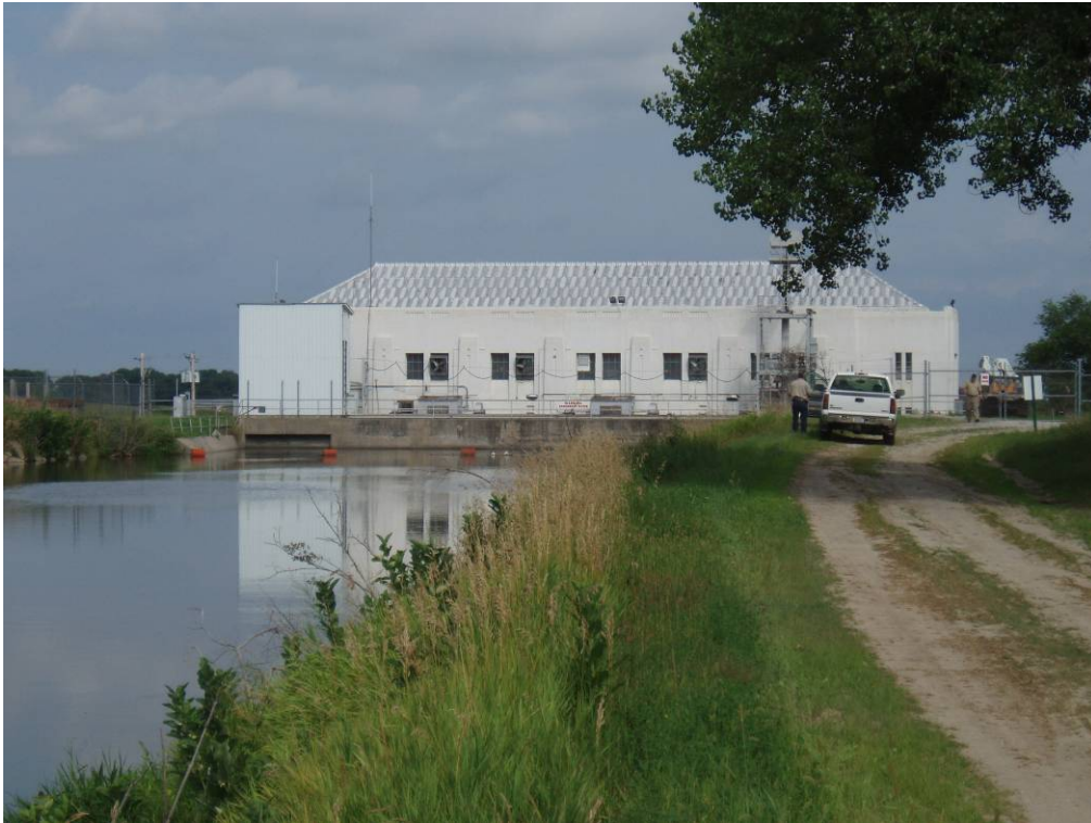
Photo 4-21. View of the upstream face of the Monroe Powerhouse.
