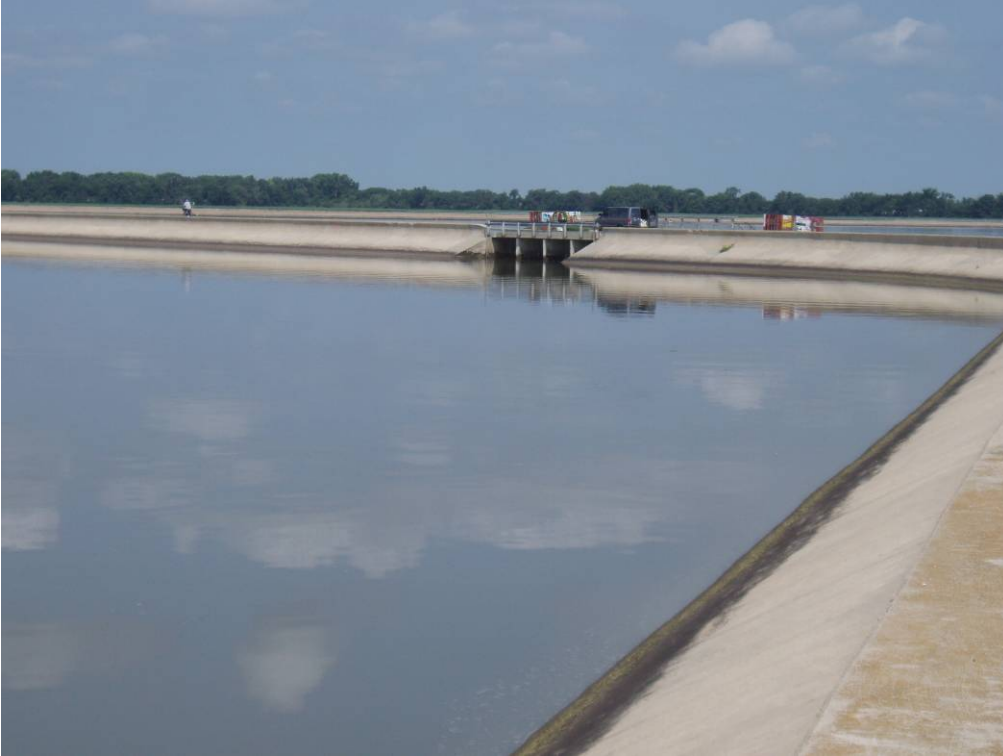
Photo 4-30. View from Lake Babcock to Lake North showing the dike that divides the two regulating reservoirs and the control structure that connects them.
