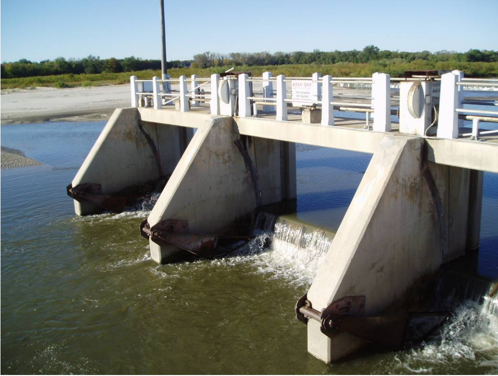
Photo 4-6. Downstream face of the Sluice Gate Structure.
