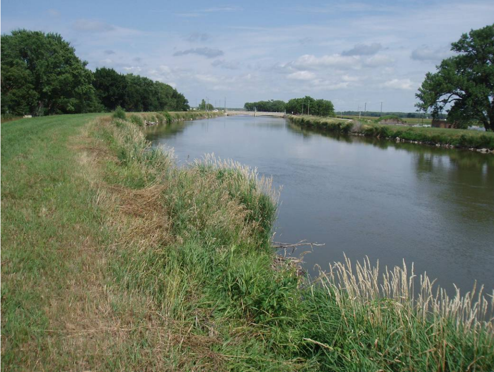
Photo 4-18. View of the Upper Power Canal in Genoa.
