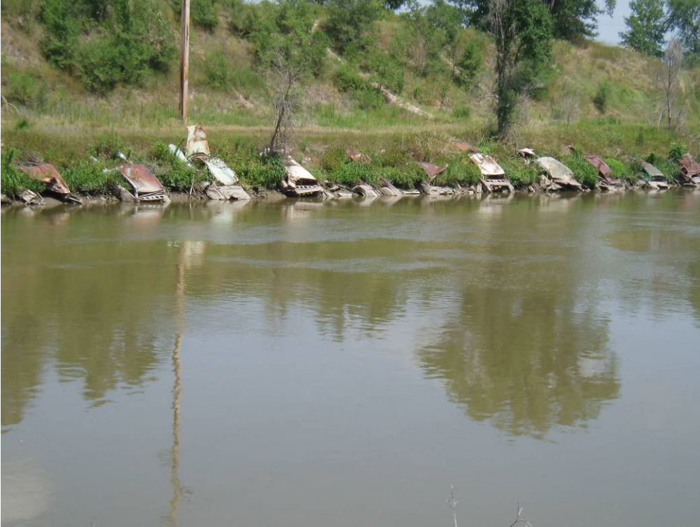
Photo 4-40. View of the unique shoreline stabilization along the Tailrace Canal.
