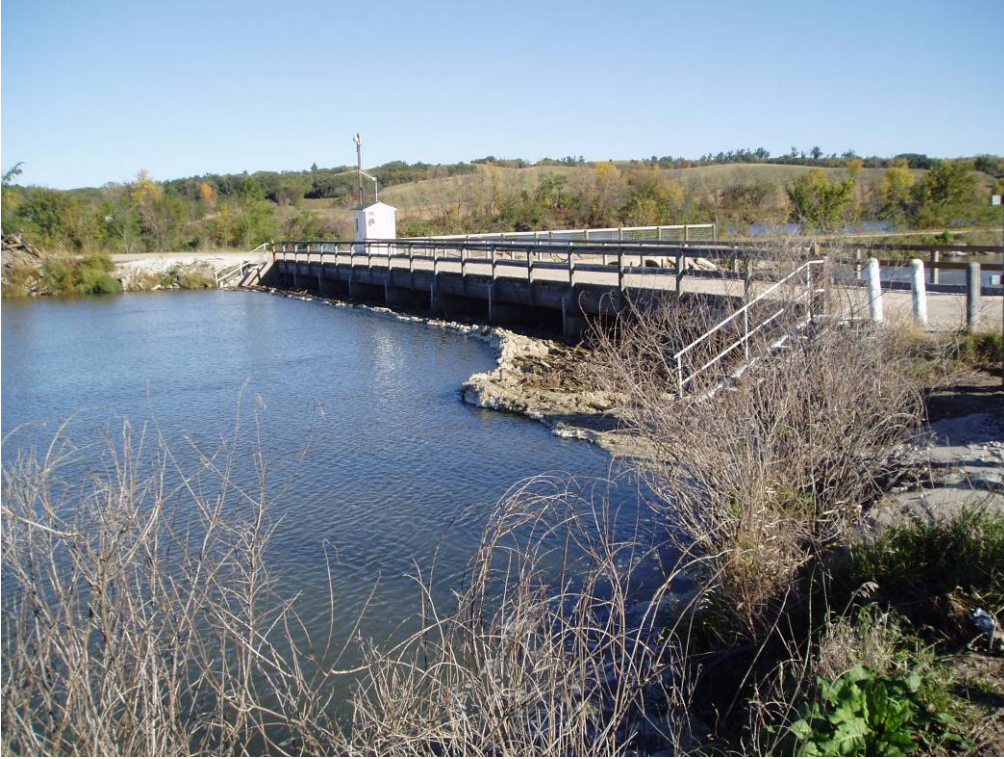
Photo 4-15. View of the Skimming Weir from upstream.
