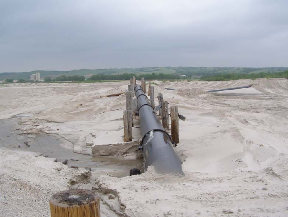
Photo 4-14. Typical view of the North Sand Management Area.
