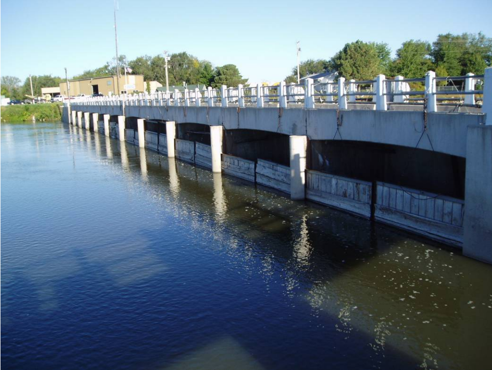
Photo 4-3. View of the Intake Gate Structure from the Sluice Gate Structure.
