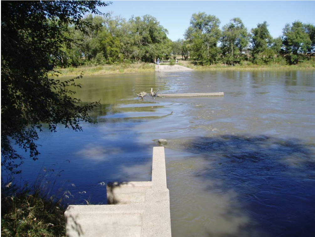
Photo 4-25. Unique turbulence created by the submerged Sawtooth Weir.
