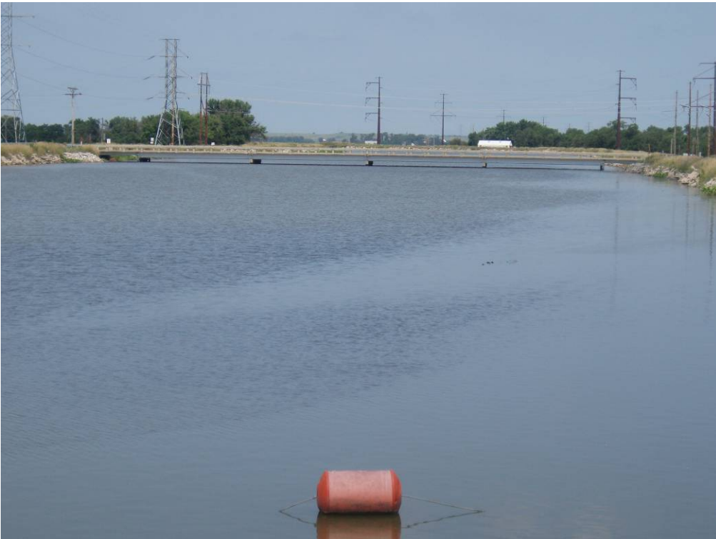
Photo 4-32. View of the Intake Canal from the Powerhouse Inlet Structure.
