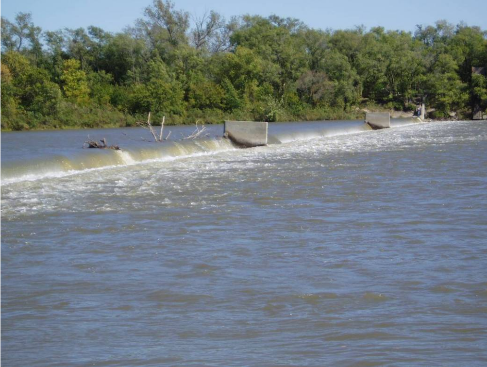
Photo 4-41. View of the Outlet Weir from the west bank.
