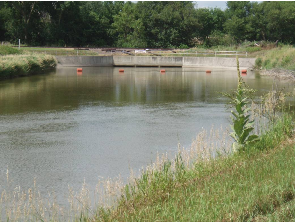
Photo 4-19. View of the approach to the Railroad Siphon at Genoa.
