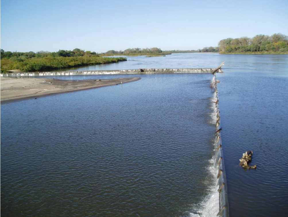
Photo 4-2. View of the Diversion Weir from the Sluice Gate Structure.
