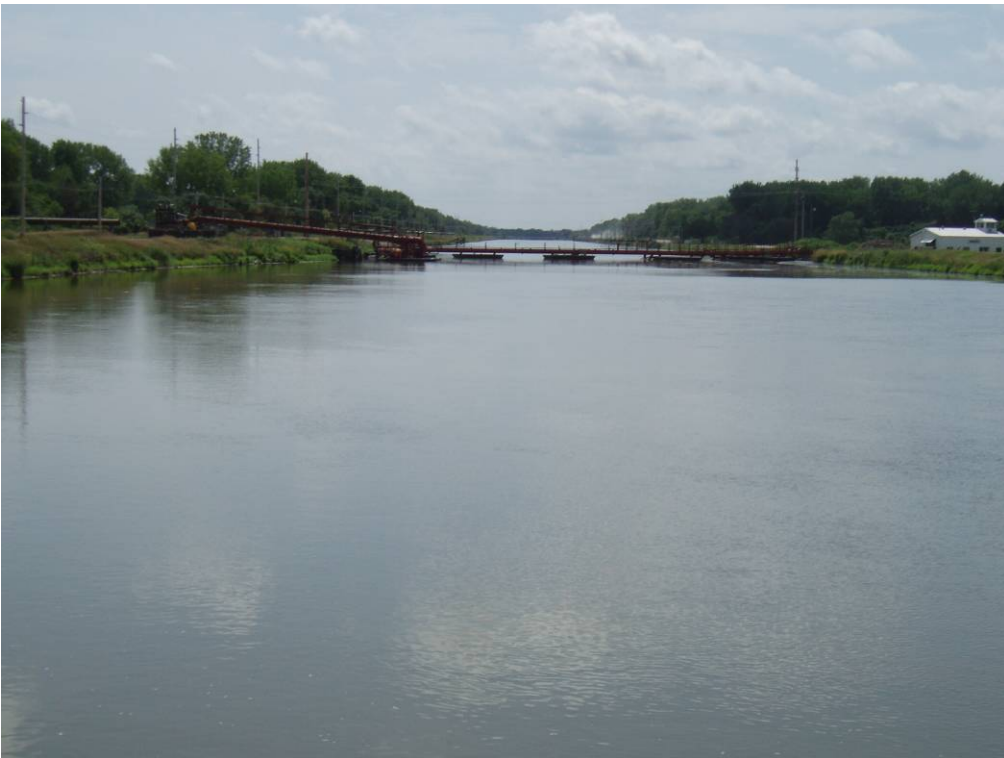
Photo 4-8. View of the Settling Basin and Hydraulic Dredge from the Skimming Weir.
