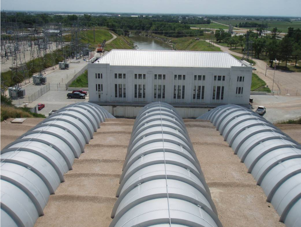
Photo 4-36. View of the Columbus Powerhouse from the Powerhouse Inlet Structure.
