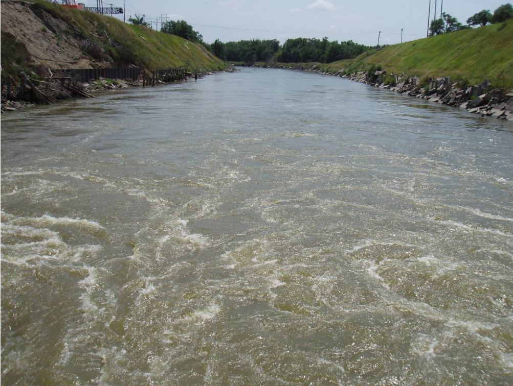
Photo 4-38. View of the Tailrace Canal from the Columbus Powerhouse.
