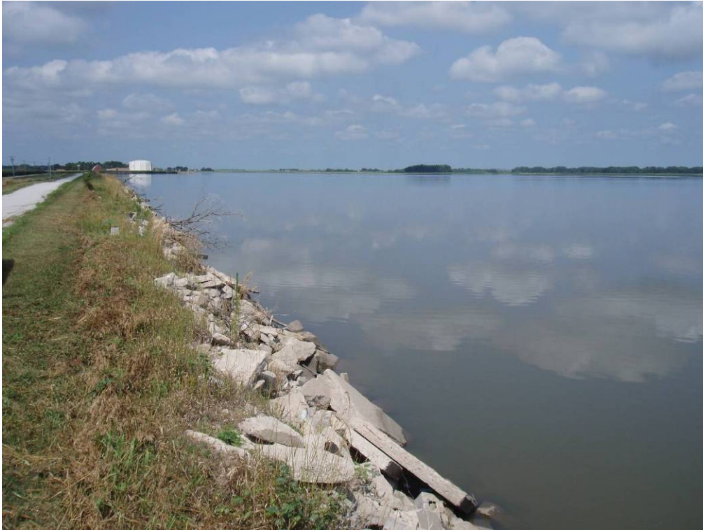
Photo 5-2. Riprap shore protection on Lake Babcock.
