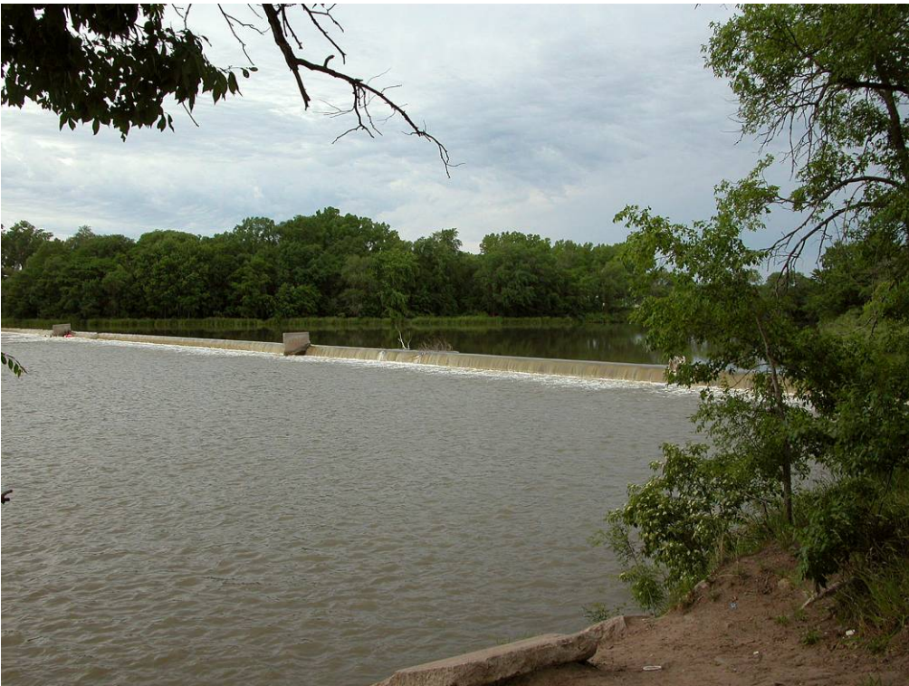
Photo 5-23. View of the Outlet Weir from the east bank.
