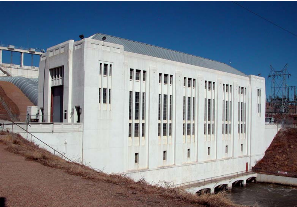
Photo 5-29. The art deco style of the Columbus Powerhouse.
