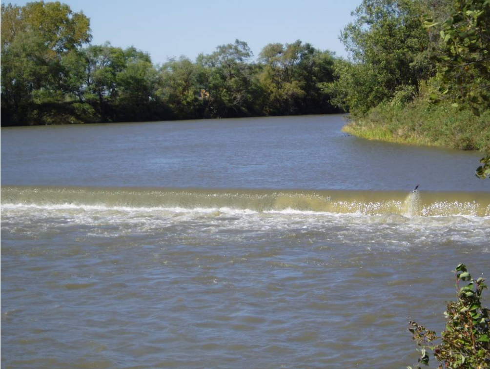
Photo 5-22. The Outlet Weir at the Platte River.
