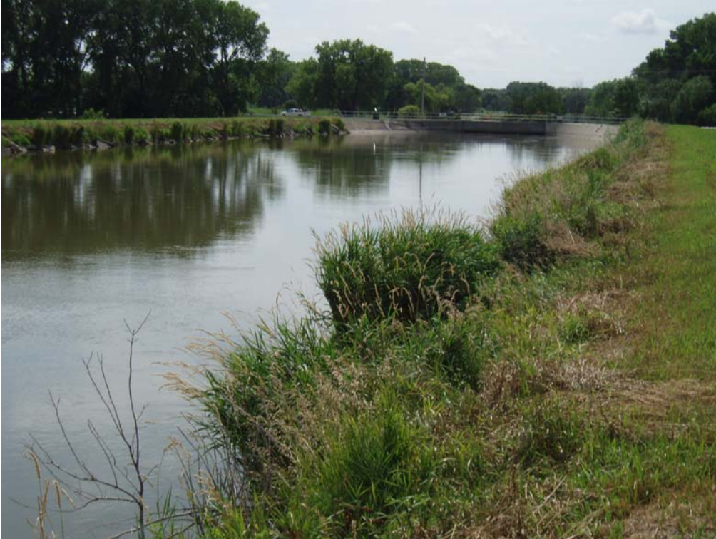
Photo 5-18. The Upper Power Canal siphon at Genoa.
