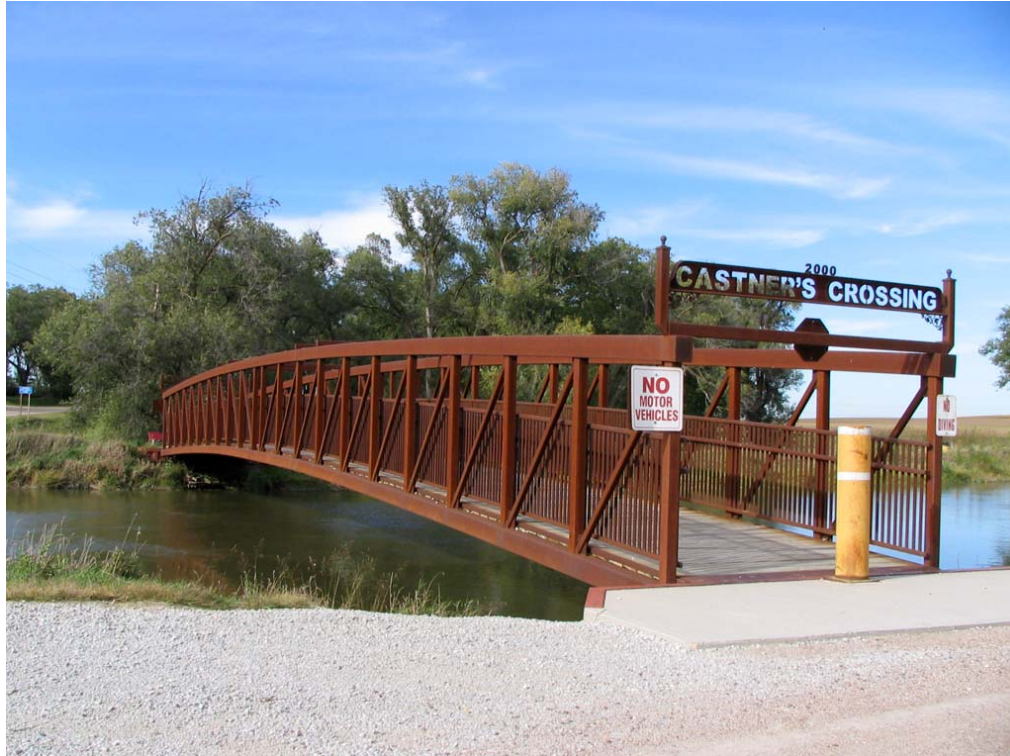
Photo 5-16. Castner's Crossing footbridge, which crosses the Loup Power Canal and connects the Two Lakes Trail and the Bob Lake Trail.
