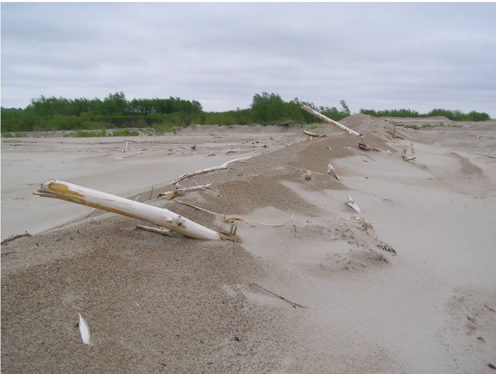
Photo 5-7. Protective berm in 2008; limbs and branches stabilize sand.
