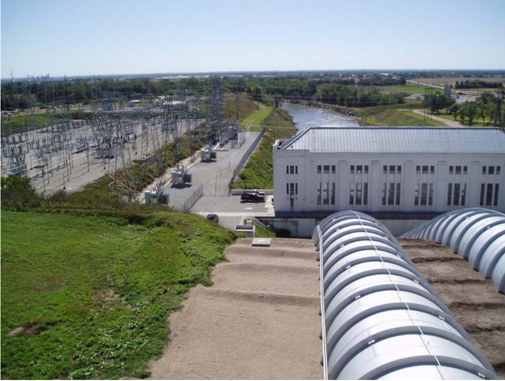
Photo 5-28. The Columbus Powerhouse and substation.
