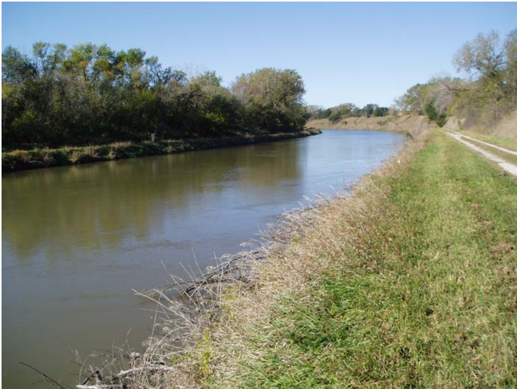
Photo 5-17. View of the Upper Power Canal.
