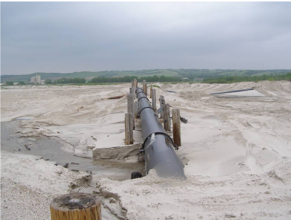
Photo 5-9. Discharge pipe extension to divert water around berm in 2008.
