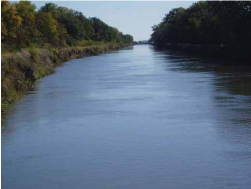
Photo 2. Typical view of the Upper Power Canal.
