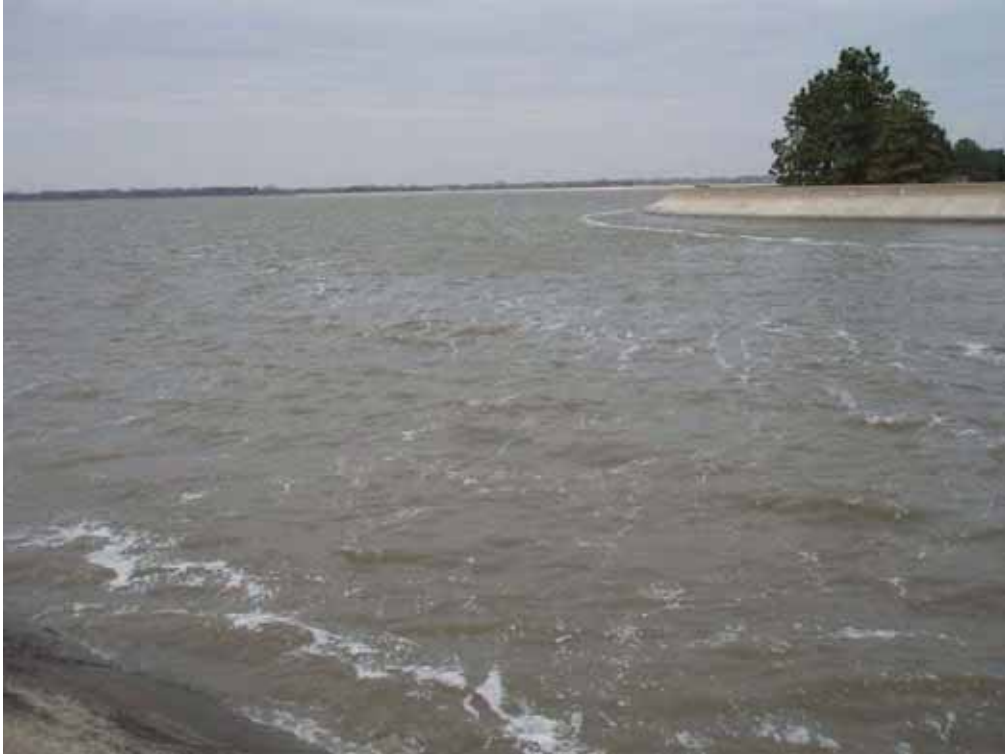
Photo 4. View of Lake Babcock from the south dike at the outlet.
