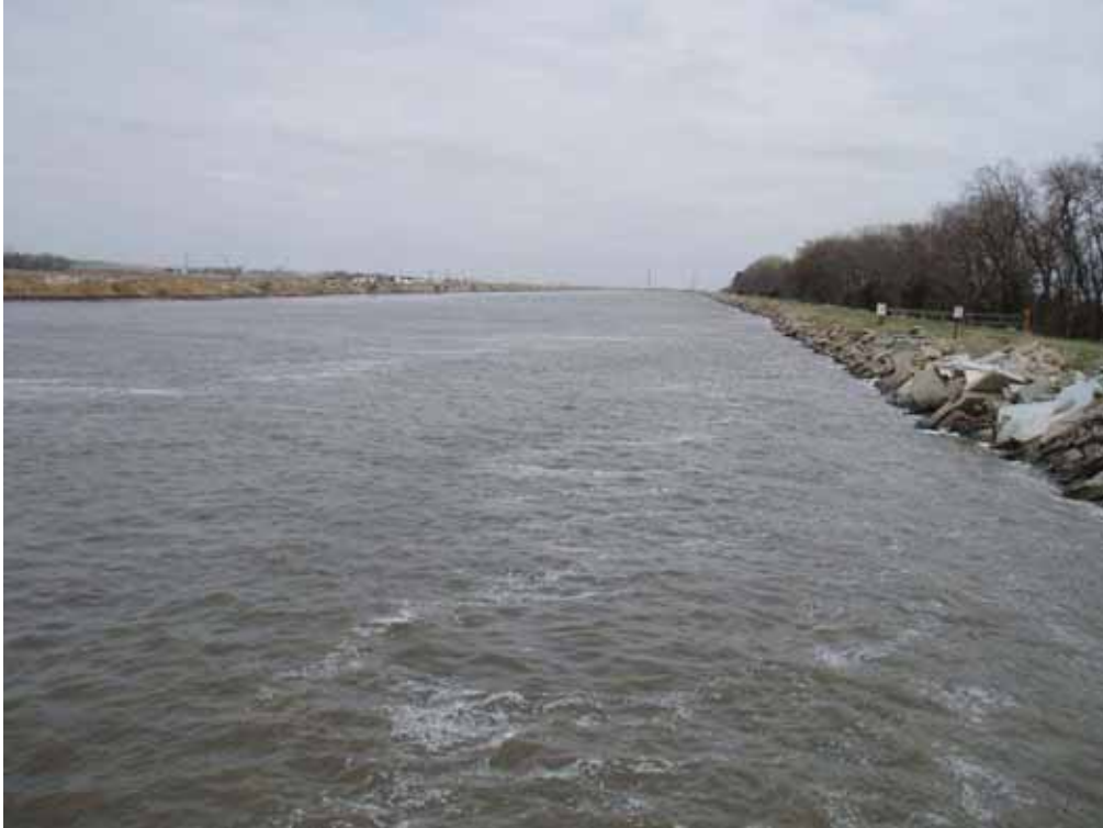
Photo 6. View of the Intake Canal as it exits Lake Babcock.
