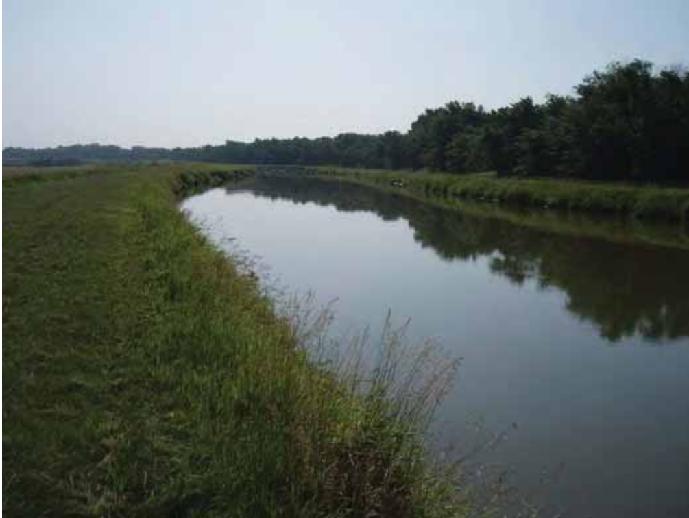
Photo 3. Typical view of the Lower Power Canal.
