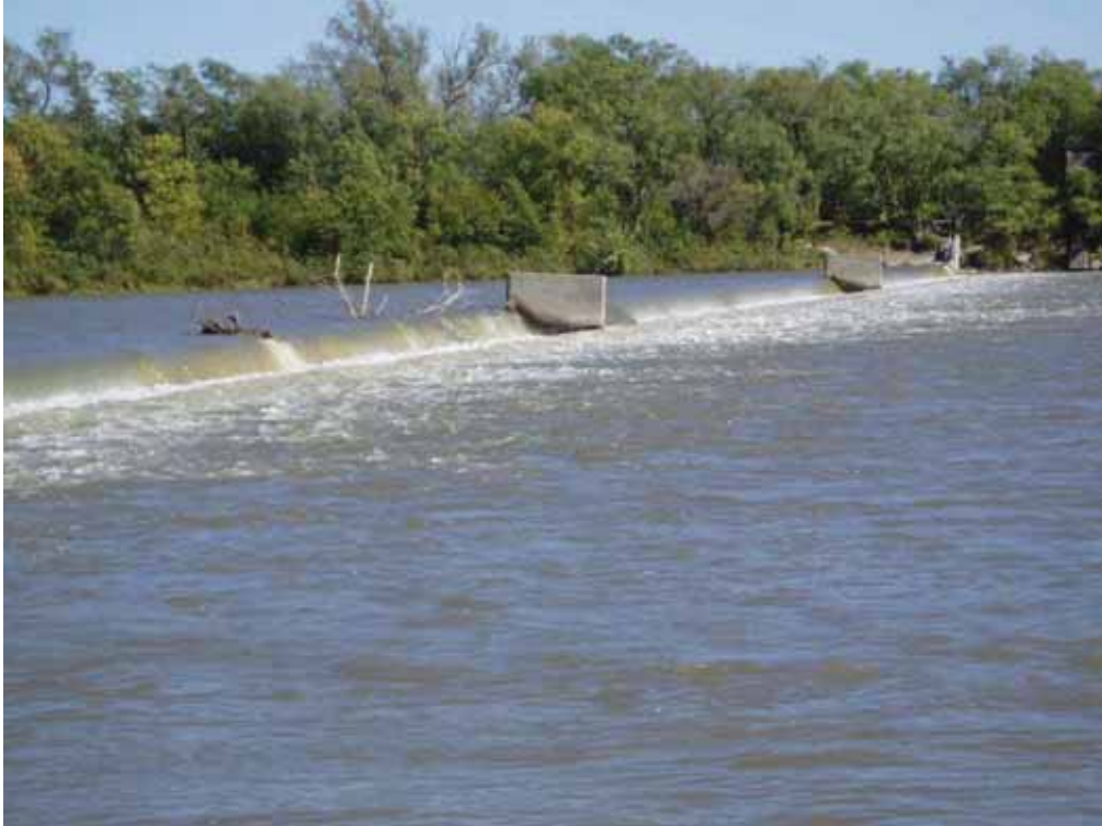
Photo 8. View of the Outlet Weir from the west bank.
