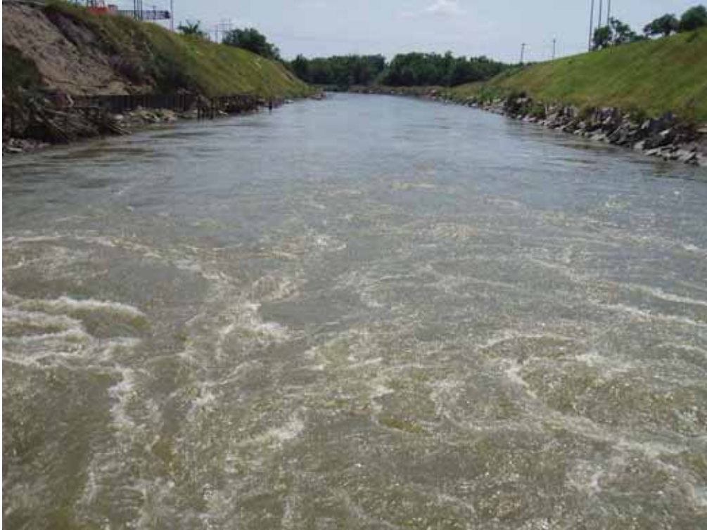
Photo 7. View of the Tailrace Canal from the Columbus Powerhouse.
