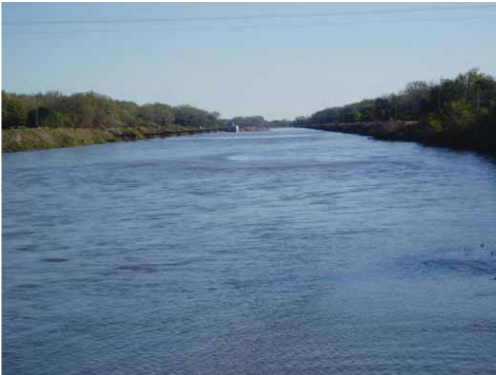
Photo 1. View of the Settling Basin from the Project Headworks.
