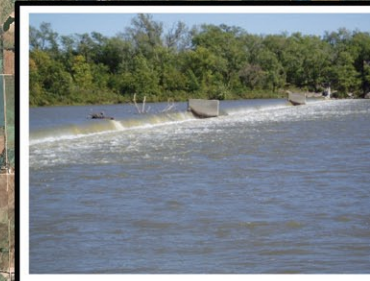
Outlet Weir at Platte River
